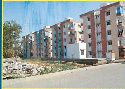
DUHS Employees Apartments
