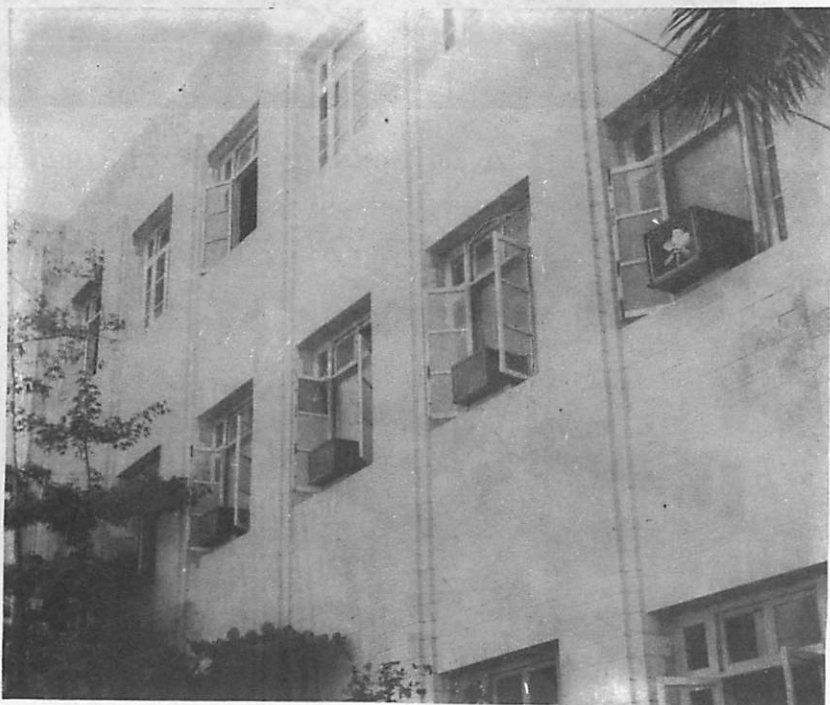
INSTALMENT OF AIR CONDITIONERS IN THE DISSECTION HALL
